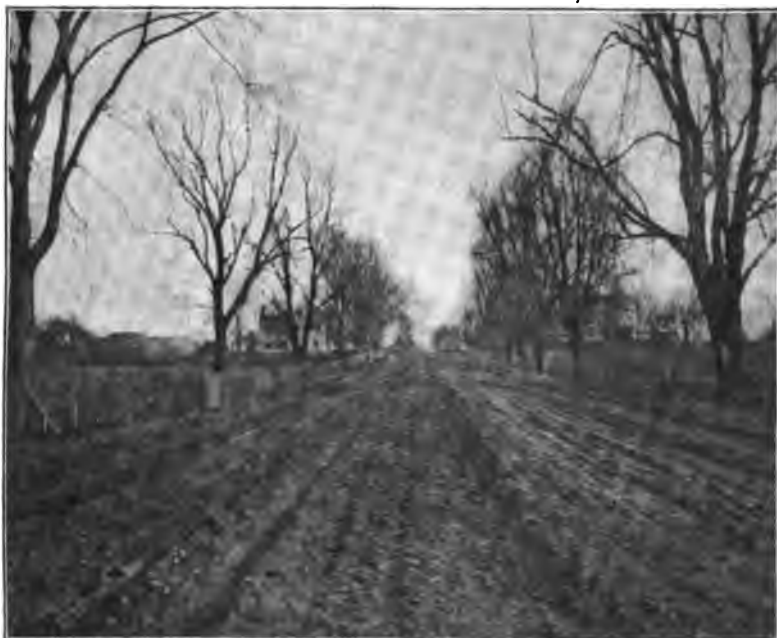
Bordentown and Crosswicks turnpike, Burlington Co., before completion.
